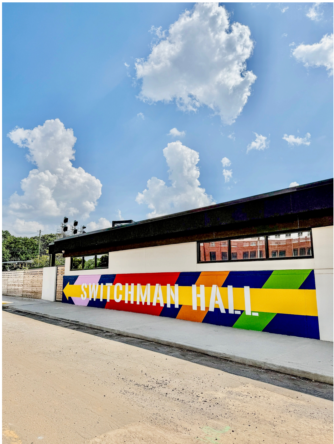
Terminal South is a vibrant adaptive reuse project in Peoplestown, located steps from the Atlanta BeltLine and the future terminus of MARTA's Rapid A-line at 1161 Ridge Avenue SW, Atlanta, GA 30315 . What began as two vacant warehouses is transforming into a community hub.
